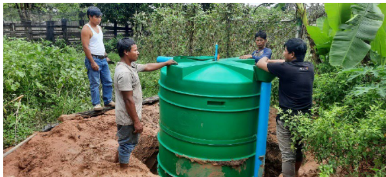
Figure 3: A biodigester producing gas from buffalo manure, used to heat-pasteurize milk
